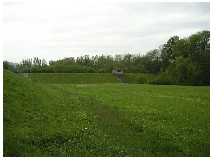
Fig. 4. Example of a Hydraulic Flood Retention Basin (type 1) in Kutzmühle (Neuenburg, Baden) on 8 May 2006.
