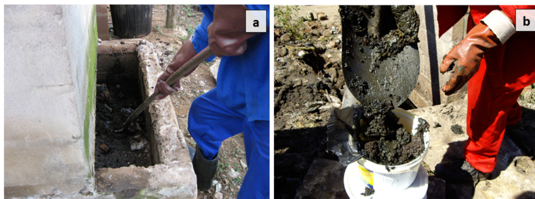
Fig. 2. Procedures of pit emptying in the eThekweni municipality (a) and sampling (b).
