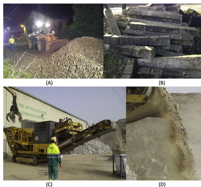
Fig. 1. (A) Ballast waste generation in the renewal of ballast track left. (B) Out-of-service concrete sleepers. (C) Crushing procedure to obtain the recycled aggregates. (D) Crushing procedure detail.
