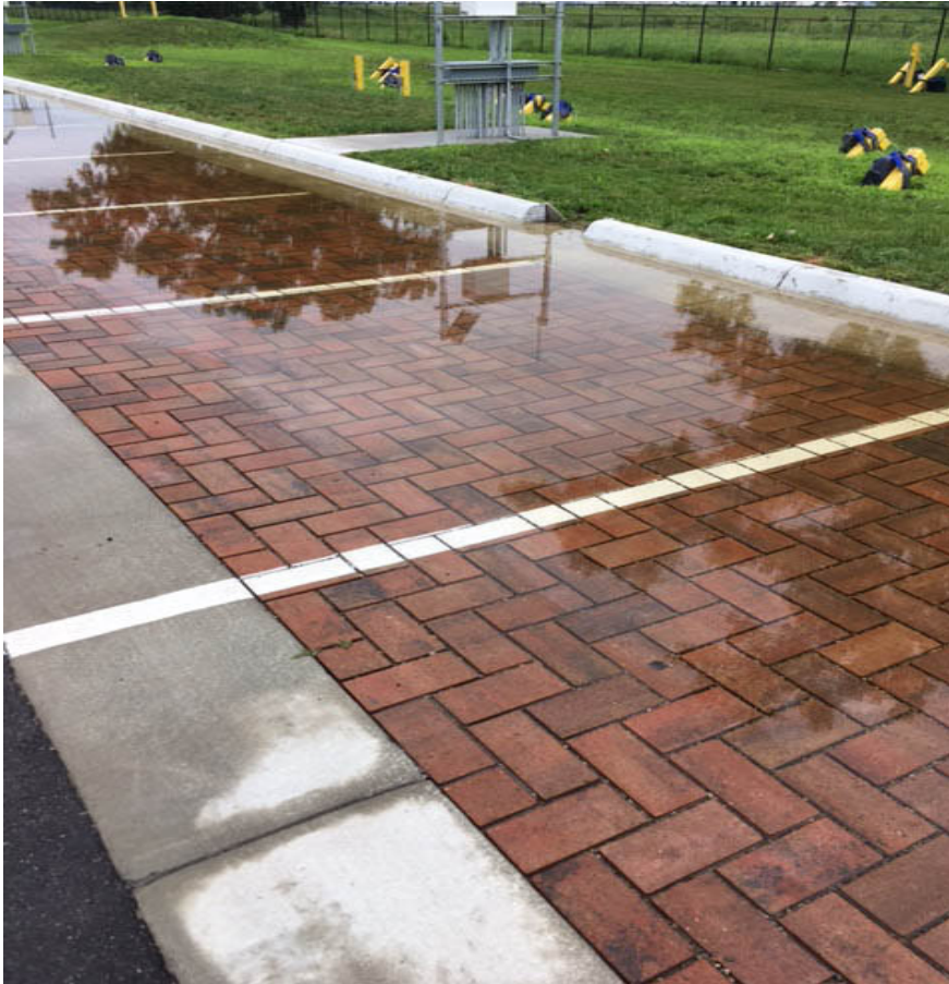
Figure 5 Standing water over PICP section after progression of clogging
