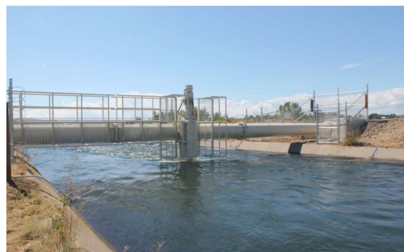
Fig. 2. Structure to support testing of a turbine that produces electricity from flowing water. Instream Energy Systems of Vancouver, B.C., built this structure over the Roza Canal in the Yakima Basin in Washington State to support testing of a turbine that produces electricity from the flowing water. (Used with permission of Instream Energy Systems Corporation).
