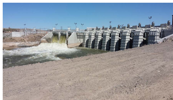
Fig. 7. Eight siphon-type Kaplan turbines. The units were installed by North Side Canal Company in Idaho, United States, in 2015. The site has a 6 m of head and a total of 1.28 MW installed capacity. (Used with permission of A Hansten of North Side Canal Company).
