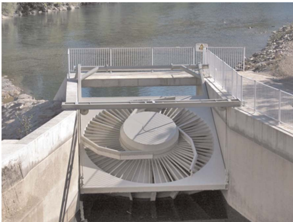
Fig. 9. A 410-kW very-low-head turbine unit in the Tarn River, Millau, France. (Used with the permission of MJ2 Technologies S.A.S.).
