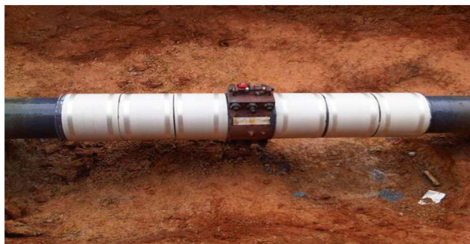
Fig. 10. Crack repair using crack arrestors [163].
