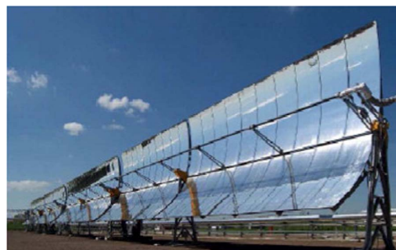
Fig. 3. CSP plant from the study of Piemonte et al. [62]: solar parabolic mirrors and receiver tube (Source: [62]).
