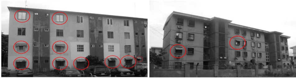
Fig. 20. Residential buildings in Abuja with improvised egg-crate shading, retrofitted overhangs and reflective glazing (2014).
