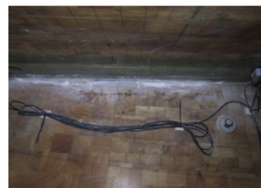
(b) Day 18- Day 20: Defect extended to 1 m x 0.05 m x 0.01 m
