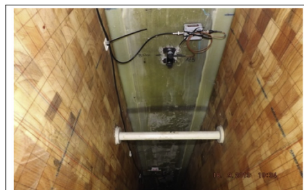
(a) AE sensors mounted between the two webs
