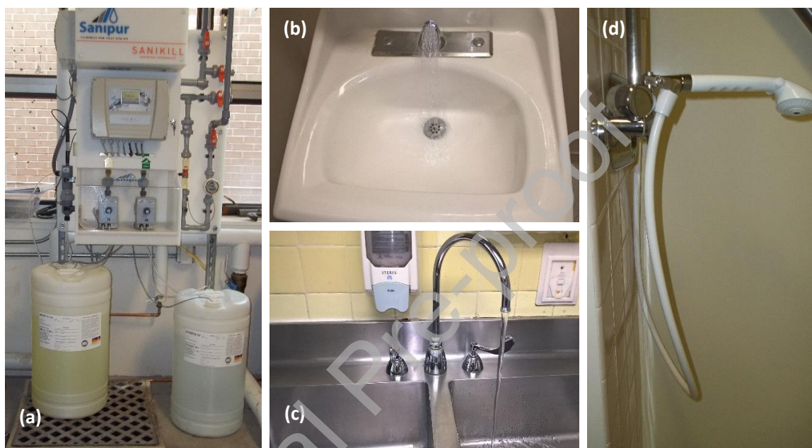
Figure 1. Photographs of (a) monochloramine on-site generator, (b) sampling site taps with double lever push button, (c) taps with traditional double lever, and (d) showerheads.
