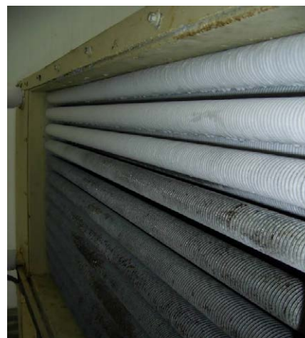
Figure 13: The photograph of evaporator at the air temperature in cold room around 1°C.
