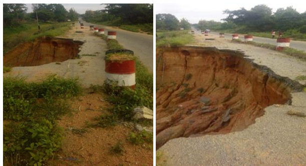
Figure 2: Failed Segment 1 at Ifon in Ondo State, showing (a) collapse pavement structure (b) eroded foundation soil and destroyed buried cables and utilities by erosion
