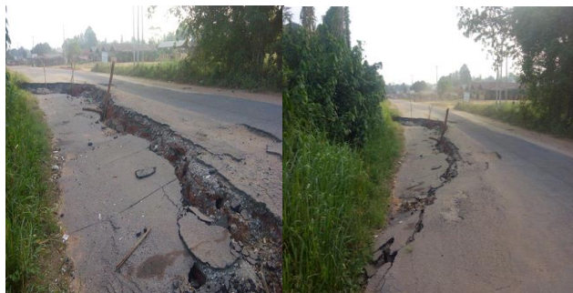
Figure 3: Collapsed Pavement Structure along Owan – Uyere Highway, representing Failed Segment 2
