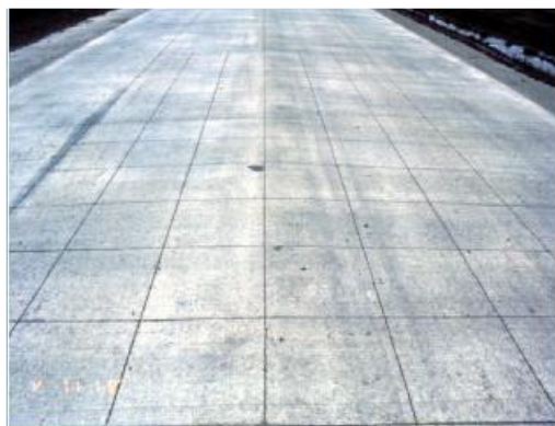
Figure 1 Ultra-Thin White topping concrete overlay with shorter Panel size
