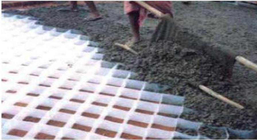
Figure 3. Laying of Cell filled concrete Pavement
