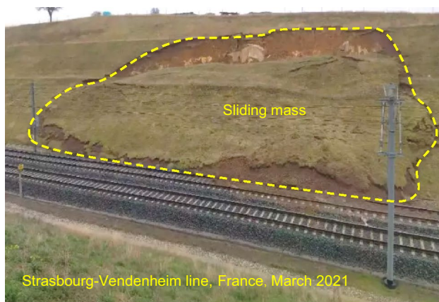
Fig. 1 An example of local instability of subgrade slopes
