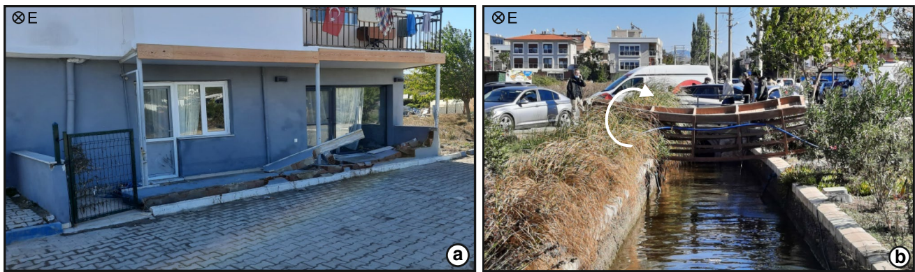
Fig. 7 a A 80-cm-high N–S-oriented wall facing the shore did not resist the tsunami destroyed walls. b A bridge on the E–W was drifted and toppled by the waves
