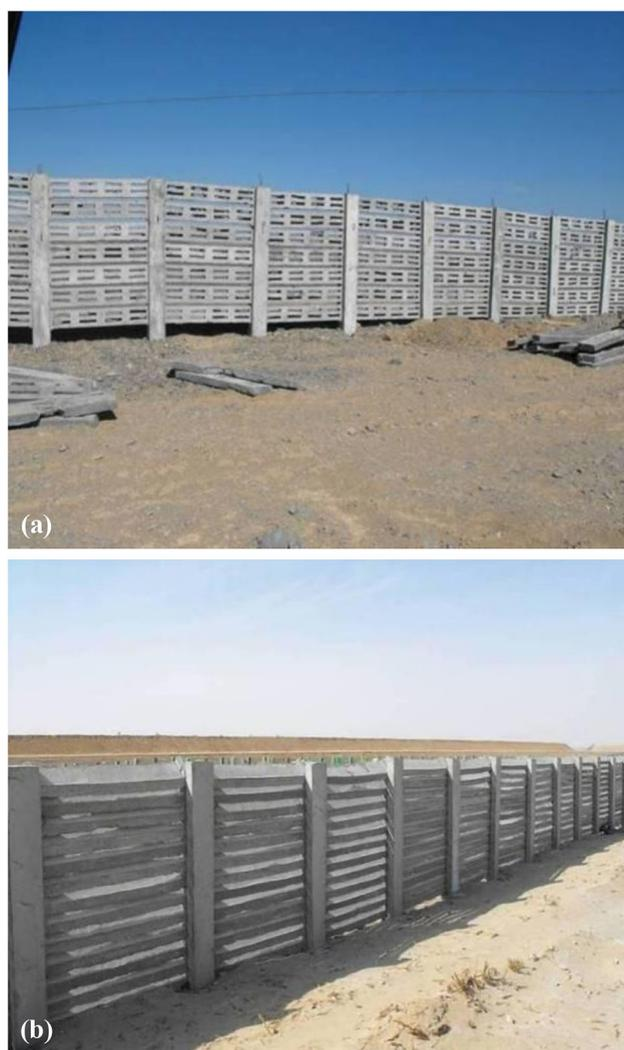
**Fig. 1** Photographs of inserting-plate sand-retaining fences: **a** SIP and **b** OIP
