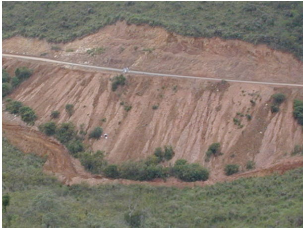
Figure 2 Illustration of an anthropogenic leak in a tropical watershed of SE Brazil. A major “leak” in topsoil and vegetation was caused by inappropriate roadwork in this mountainous region, causing a “clog” in the river downslope (not shown). A tunnel would have been a better solution. Photo reproduced with permission of André Nave.
