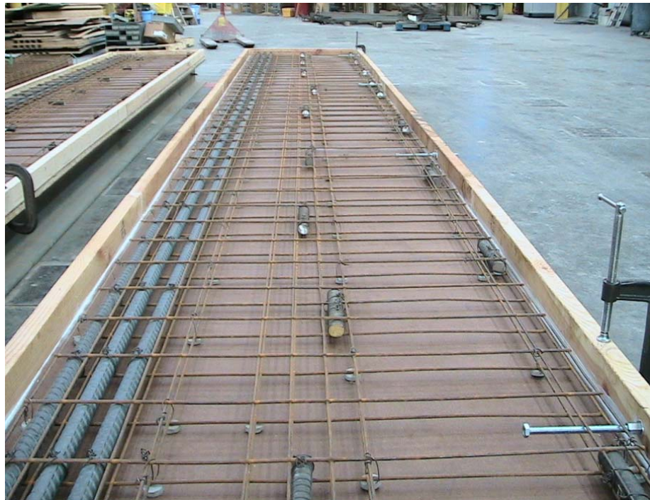
Figure 2.3 – Congested reinforcement in B36
