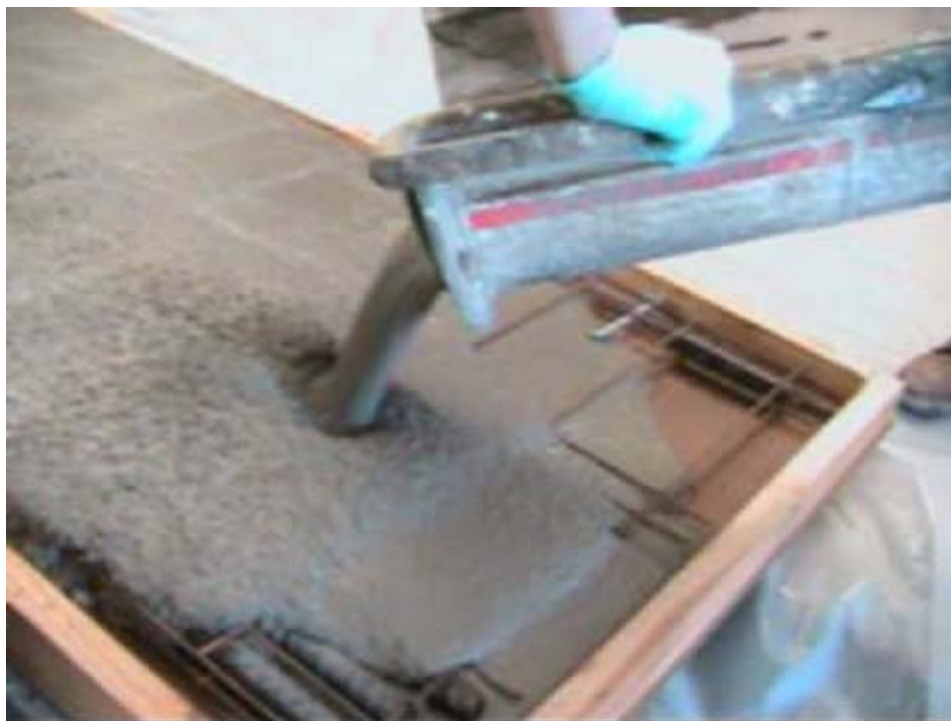
Figure 2.4 – Application of self-consolidating concrete
