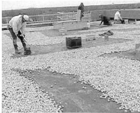
Figure 3.5 Aggregate covering [12]
