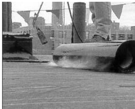
Figure 3.4 Built-up roofing membrane [12]
