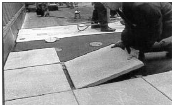
Figure 3.3 Rigid board insulation [12]
