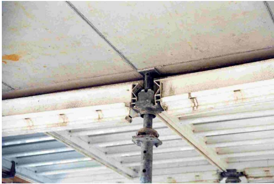
Figure 3.1 Drophead shore with removable beams and panels (courtesy of Meva)
