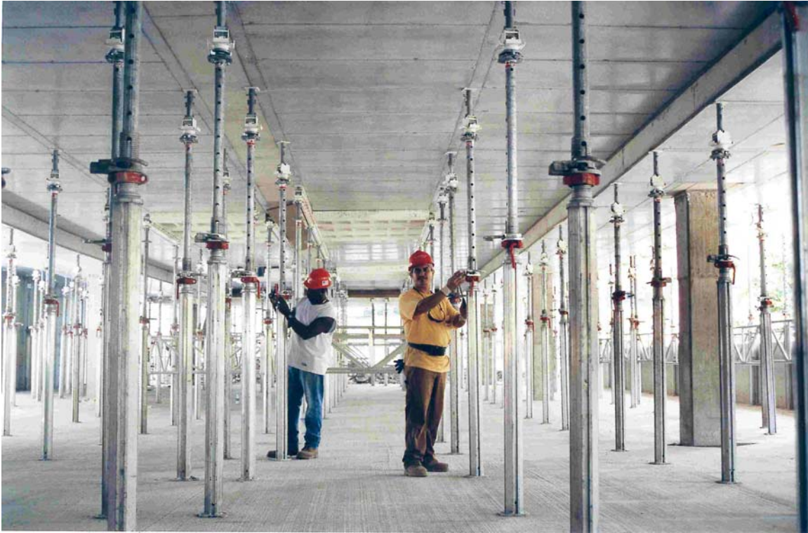
Figure 3.3 – Activation of floor slab (courtesy of Meva)
