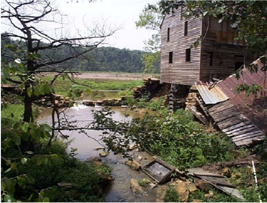
Figure 9: Yates Mill after Hurricane Fran. Notice that the shed attached to the mill has collapsed, and that the original dam was destroyed. It is believed that the dam had stood since its construction in the mid 1700s. Photo taken by Rebecca Cope; courtesy of Historic Yates Mill County Park.
