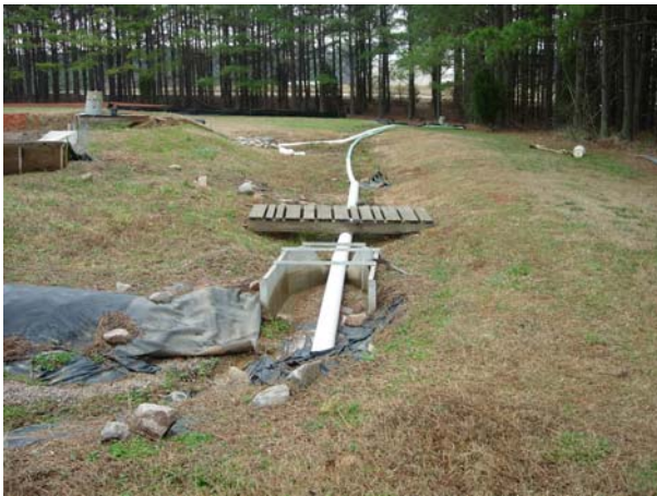
Figure 2.5: The pipe leading to the woods carries the drained water, while the channel carries the water exiting through the section cut from the wooden gate.
