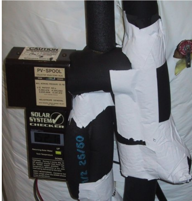
Figure 4.5 Additional Insulation Applied to the SDHW System Controls
