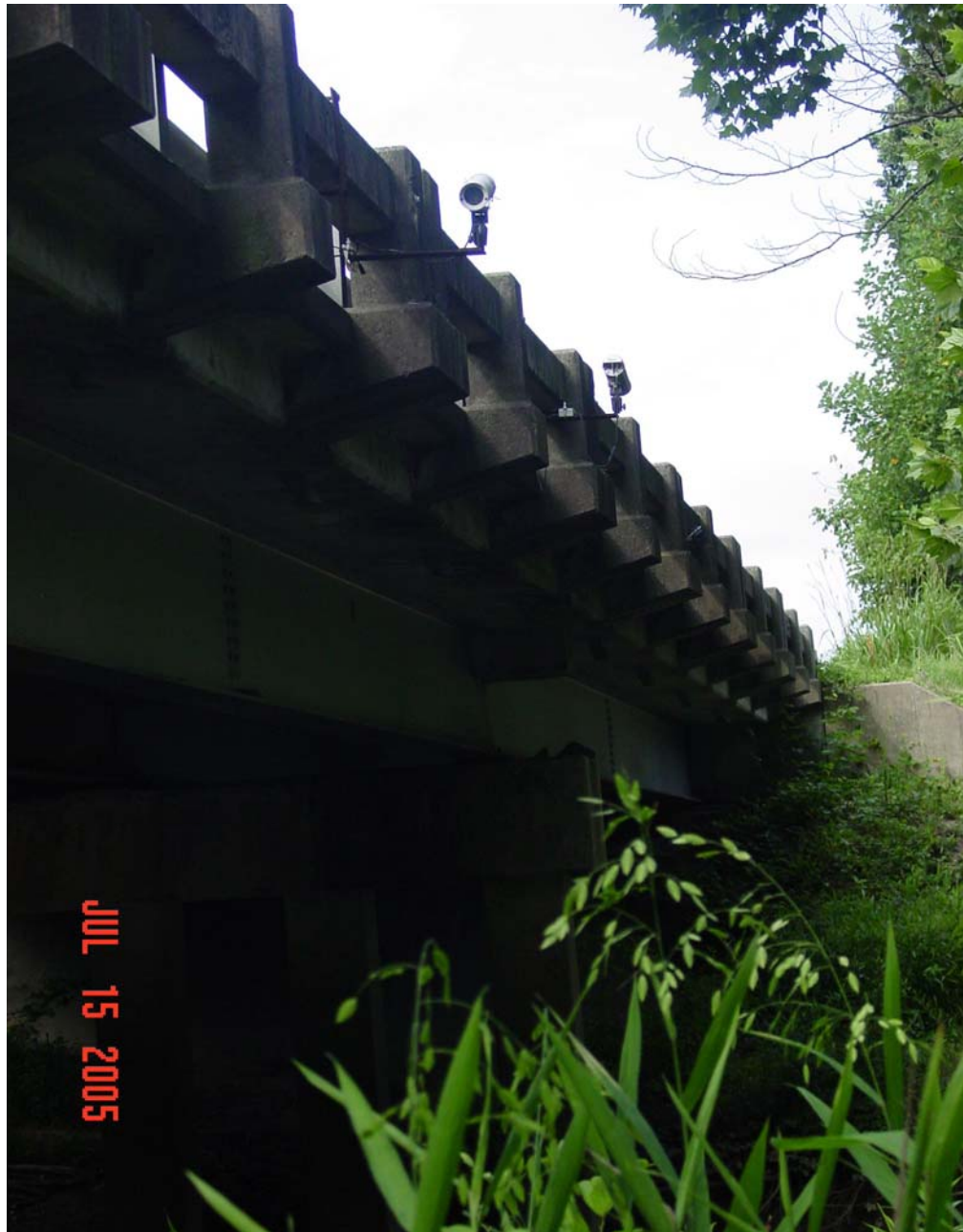
Figure 6. Cameras mounted on the north side of the southbound bridge.
