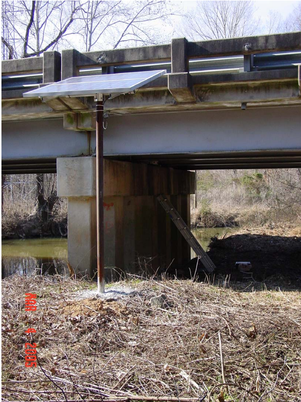
Figure 9. Solar panels installed in the open median of the NHC bridge.
