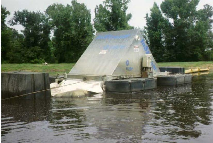
**Figure 5. InStream™ Water Unit installed in the lagoon treatment system**
