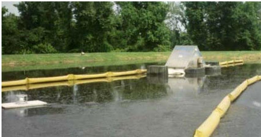
**Figure 6 . Picture showing InStream™ Water Unit, gas collection device, and two hanging baffles**
