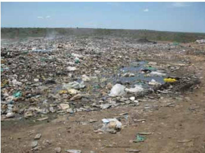
Photo 24: The wastes have not been covered with soil and occasional burning can be seen
