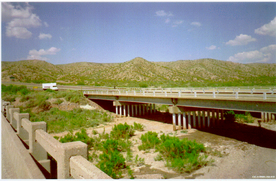
Figure 28. Source of excitation for ambient test one.
