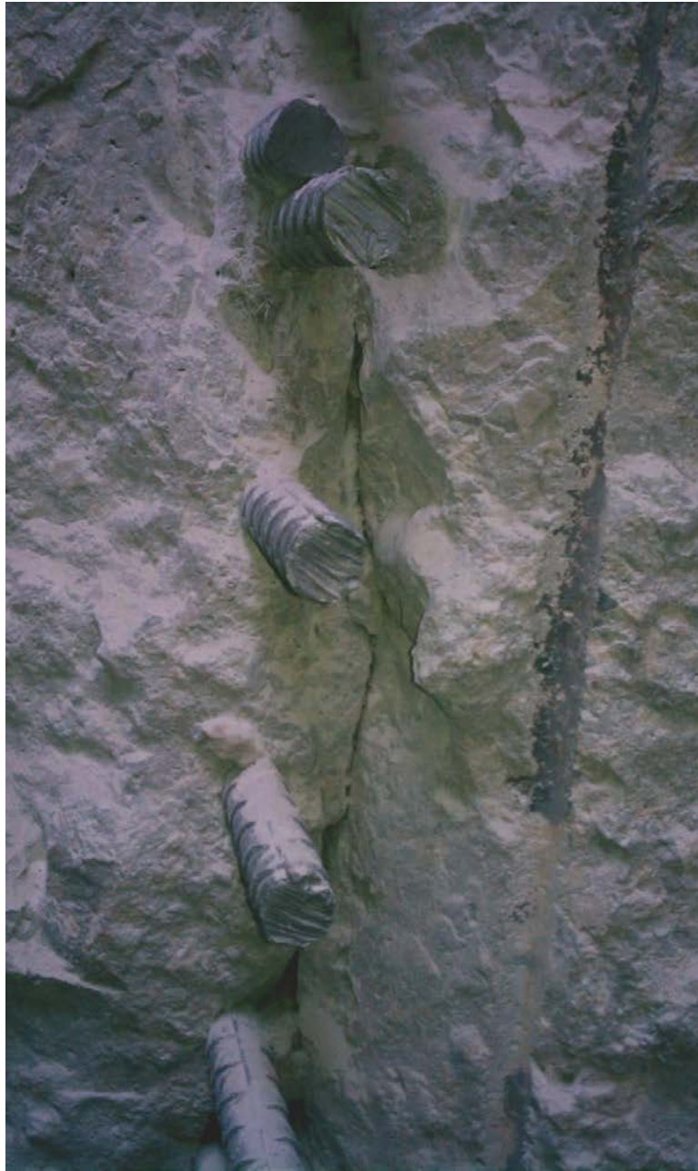
Fig. 6. Laminar cracking at reinforcements from an interface cut out by hydrodemolition [42]
