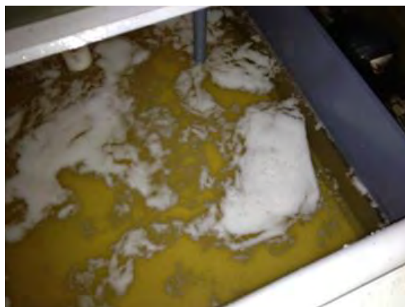
Figure 2–18 Regenerator sump showing precipitate in the desiccant, Encinitas, California (Credit: AIL Research, with permission)
