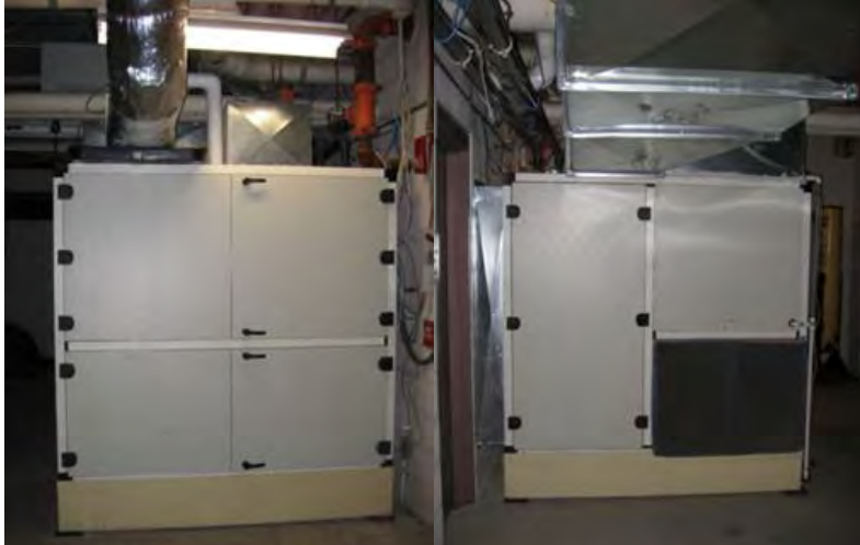
Figure 2–42 LDAC unit in the basement of the Schaefer Pool facility (Credit: AIL Research, with permission)
