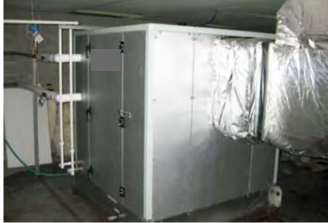
Figure 2–52 LDAC conditioner in the mechanical room of the Babbio Center (Credit: AIL Research, with permission)
