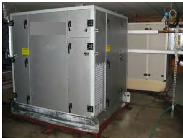
Figure 2-51 LDAC regenerator and conditioner in the mechanical room of the Babbio Center (Credit: AIL Research, with permission)
