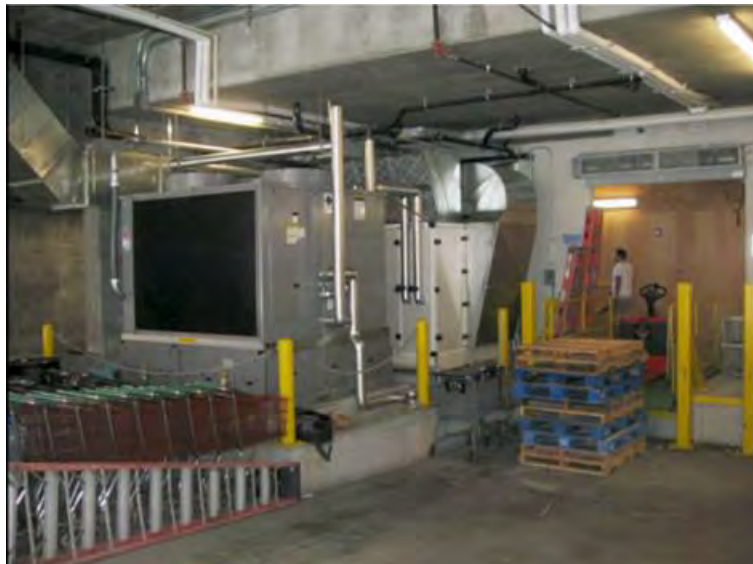
Figure 2–6 LDAC and chiller system in loading dock at Whole Foods, Encinitas, California (Credit: Jeff Miller/AIL Research, with permission.)
