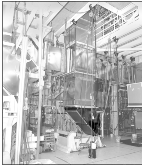
Figure 6: An LM5 upward-facing elbow enclosure installed in the NIF beam path.
