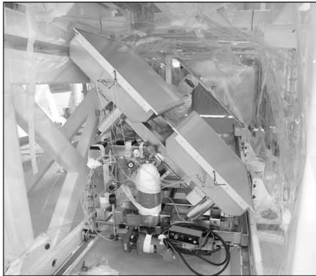
Figure 5: Removal of an LM5 LRU. Local cleaning requires the construction of local clean rooms in areas, which can be very congested.
