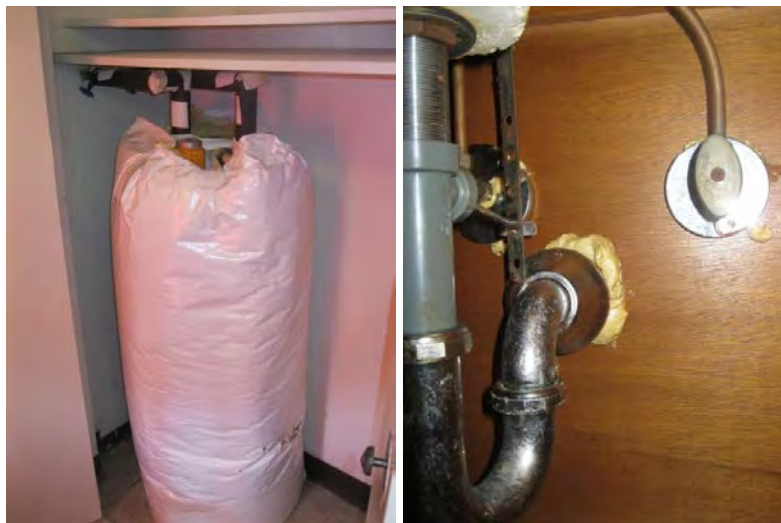
Figure 3. Electric storage water tank with insulation wrap (left) and foamed plumbing penetrations (right) at IHA
