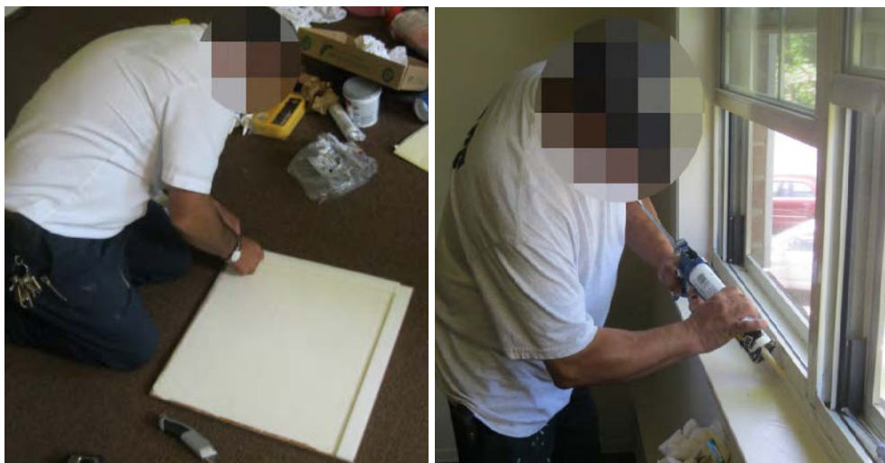
Figure 4. Installing gasket on attic hatch (left) and caulking gap around window (right) at IHA
