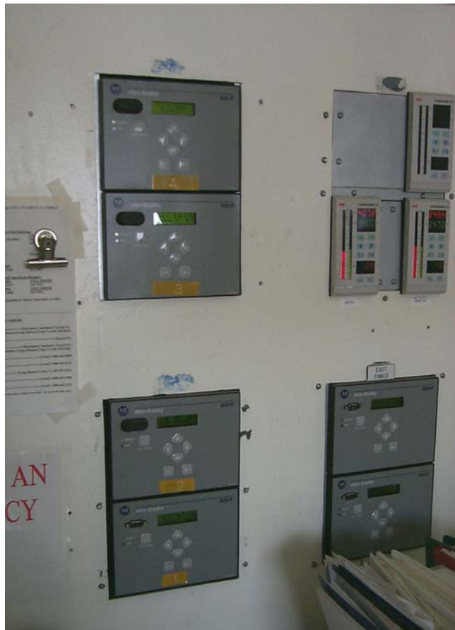
Figure 5 (PH0022) Allen Bradley Motor Protection (model 825-p)
