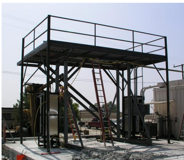
Figure 4. Reactor support framework before pilot plant assembly.
