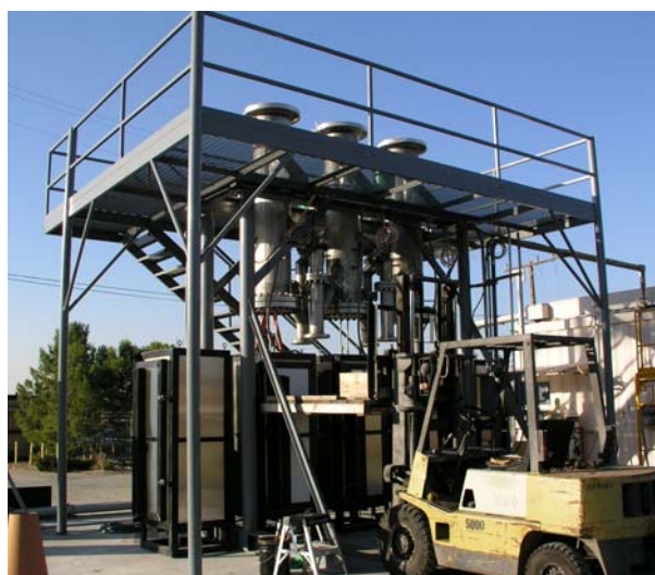
Figure 5. Reactors assembled on support framework.
