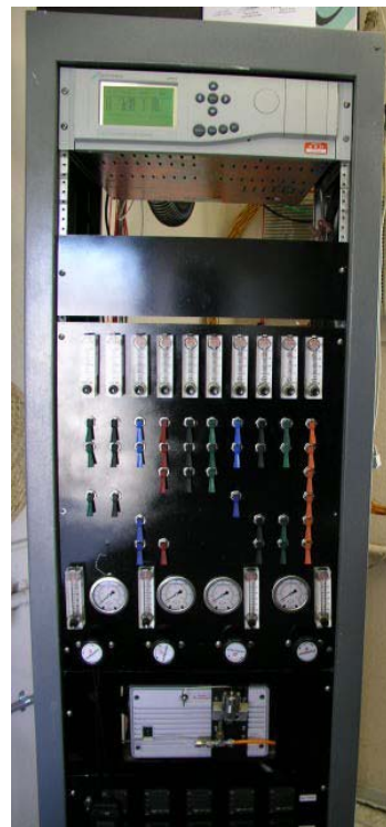
Figure 9. CEMS rack with controls for product and calibration gas flow to analyzers.
