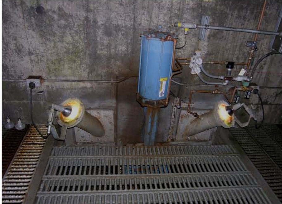
Figure 2.7. Top portion of light tubes in downstream migration channel with halogen lights installed
