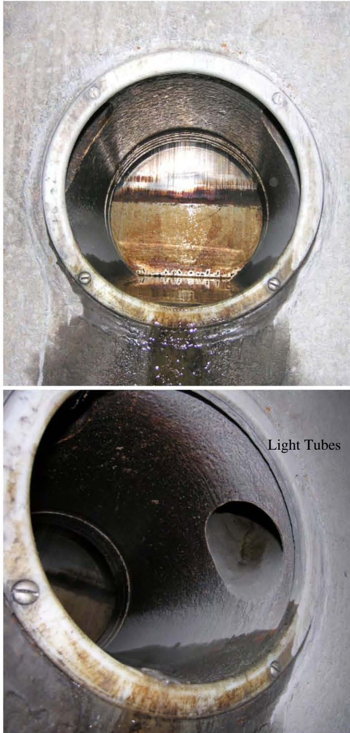
Figure 2.6. Dewatered closed orifice at north end of Gatewell 13B showing light tubes at orifice entrance
