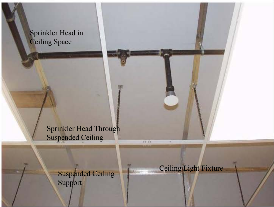
Figure 5. Existing Sprinkler System in Test Room
