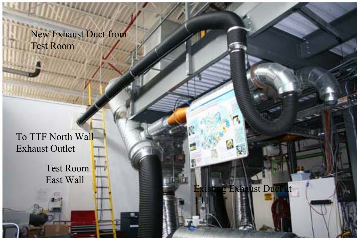
Figure 4. Exhaust Duct System of Thermal Conversion Laboratory at TTF
