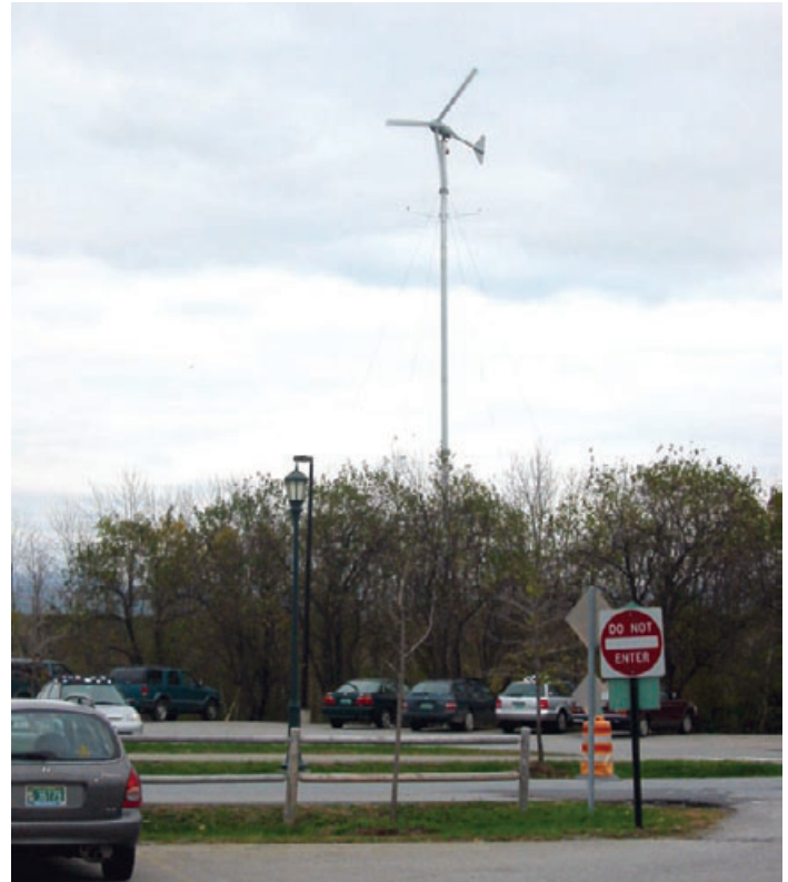
A 10-kW Bergey wind turbine installed at the University of Vermont campus in Burlington. Photo credit: Brian Killkelley
