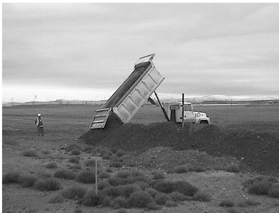
Figure 3. Dump Truck Unloading Clean Fill Material.
