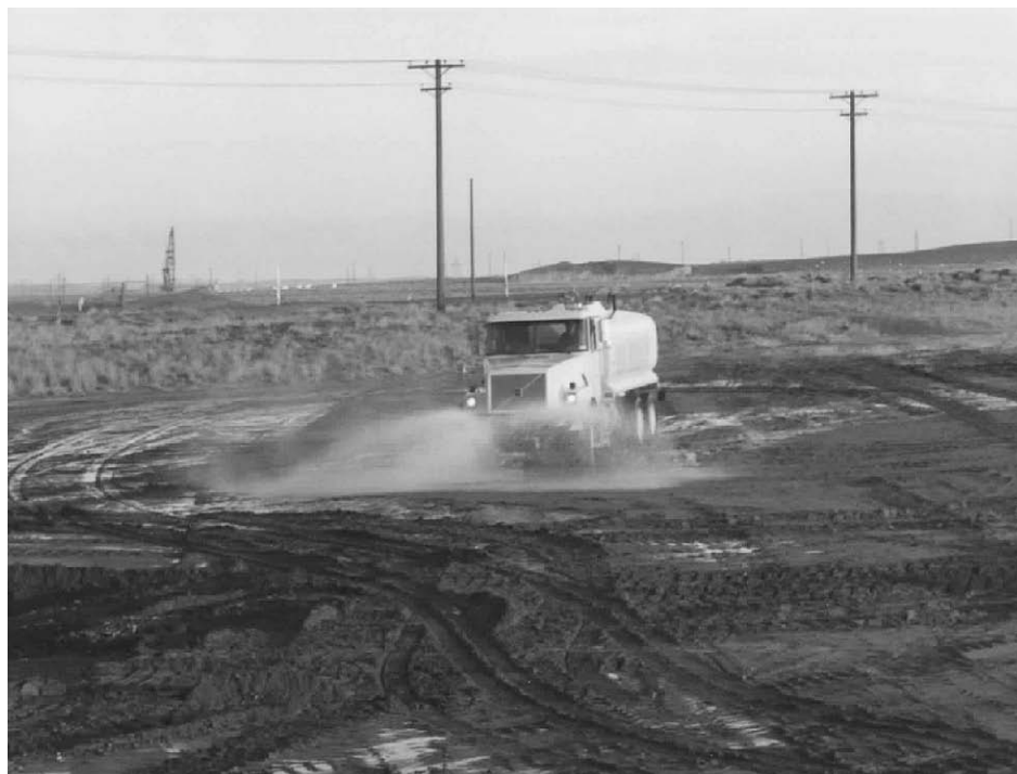
Figure 2. Water Truck Saturating Borrow Pit with Water.
