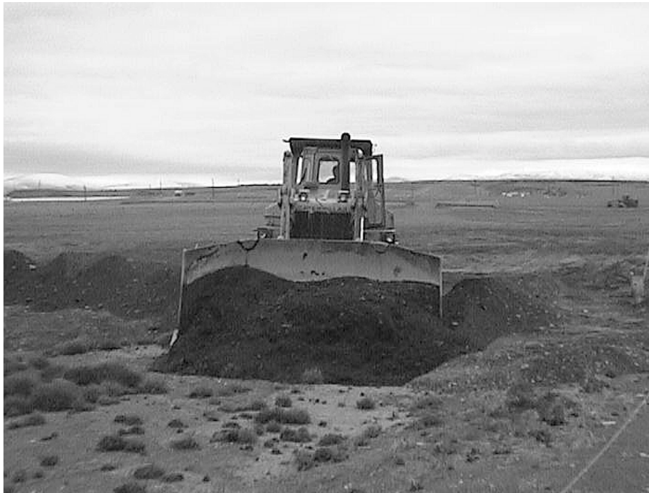
Figure 4. Bulldozer Stabilizing Clean Fill Material.
