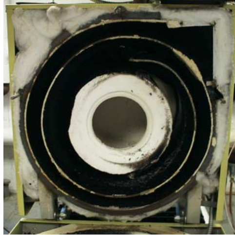
Figure 12 Boiler heavily sooted
