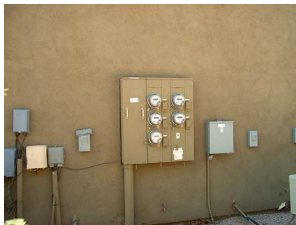
Figure 5-15. Typical apartment electrical distribution point.
