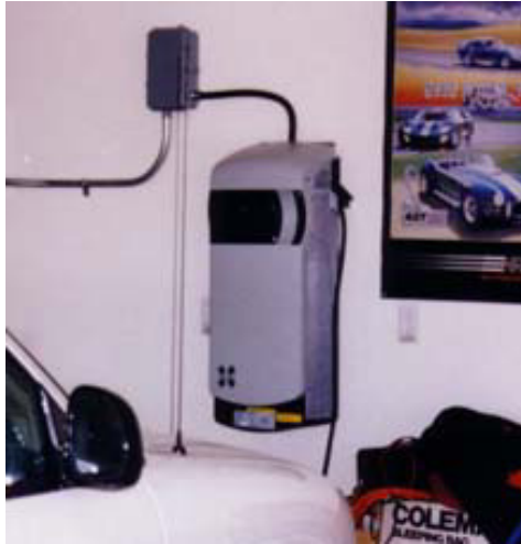
Figure 5-14. Typical Level 2 residential garage charger installation.
