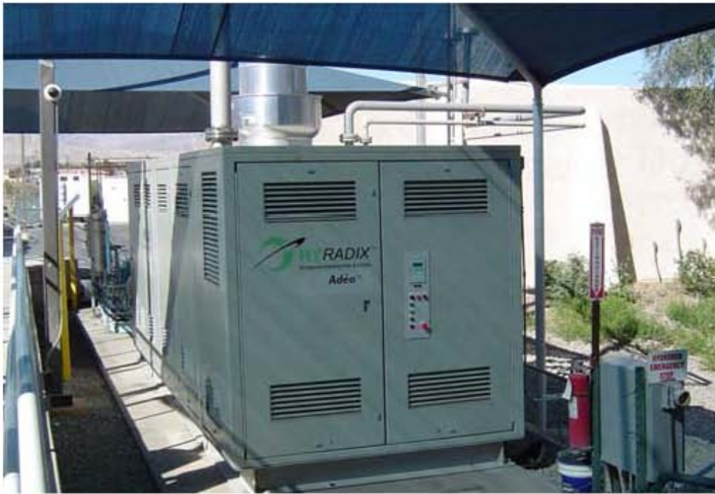
Figure 4. SunLine's HyRadix Adéo commercial reformer
