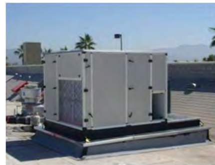
Figure 1–1. Example LDAC in a dedicated outdoor air system (DOAS) application.
