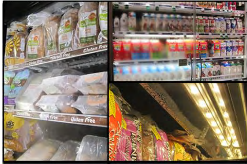
Figure 5–2. Effects of high grocery store humidity levels on refrigerated cases.
