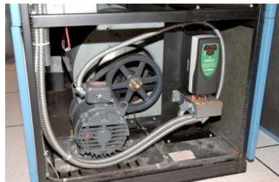
Figure 5: VFD installed.
