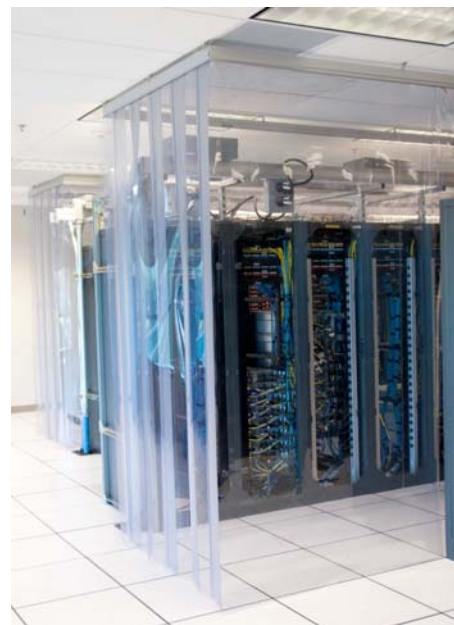
Figure 7: hot-aisle containment curtains.
