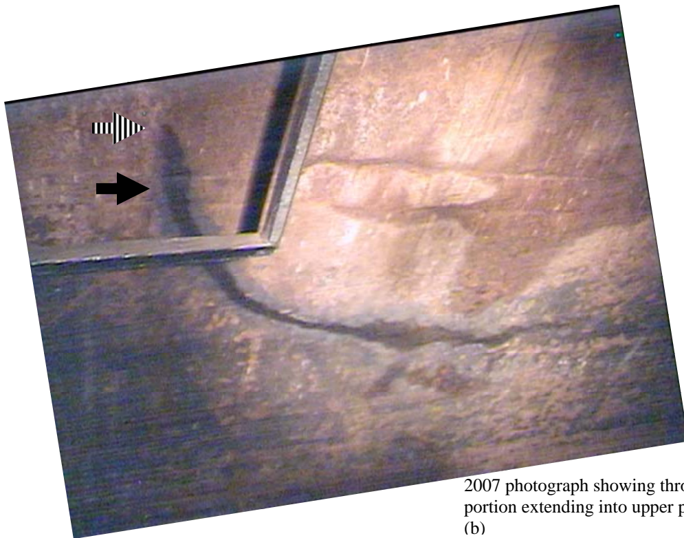
Figure 25. Bleedout photographs of crack # 6 (a) 2002 and (b) 2007.
