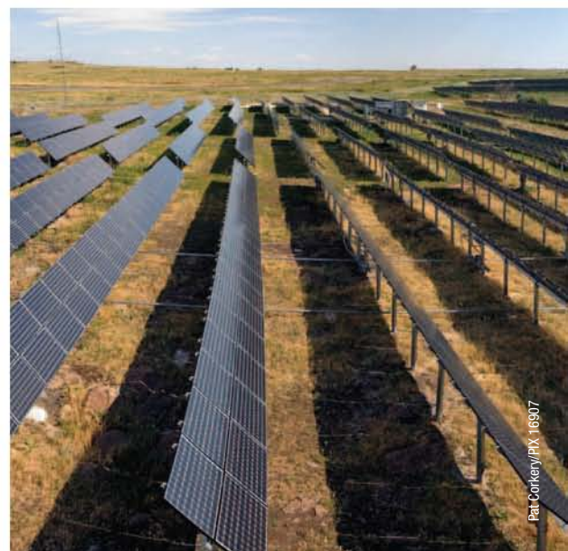
NREL's 750-kW solar system on the Mesa Top
