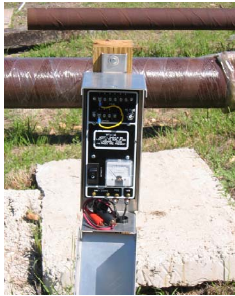
Figure 10. Details of CP rectifier installation
