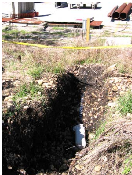
Figure 11. Magnesium anode in place before covering
