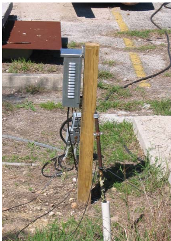
Figure 9. CP installation at the north end of test pipeline
