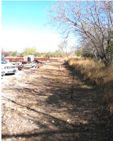
Figure 8. Test pipeline “right of way” viewed from south to north. Ground rods are set 15 feet to the right of the pipeline in this view.
