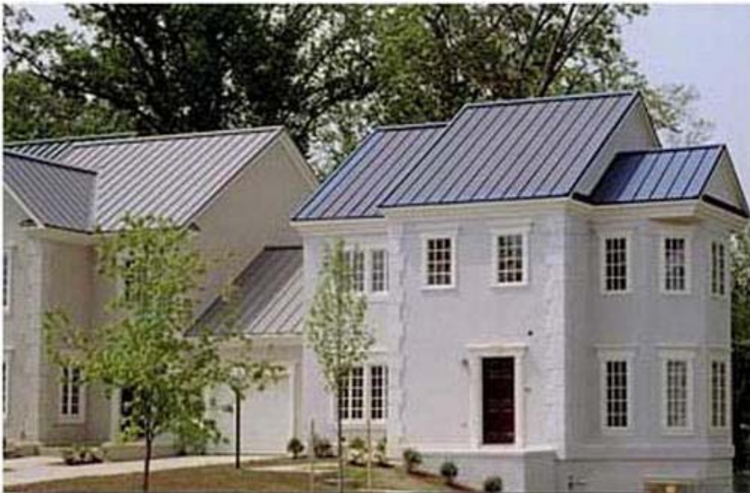
Figure 5. This 1.5-kW solar roof appears almost identical to conventional roofing material.
