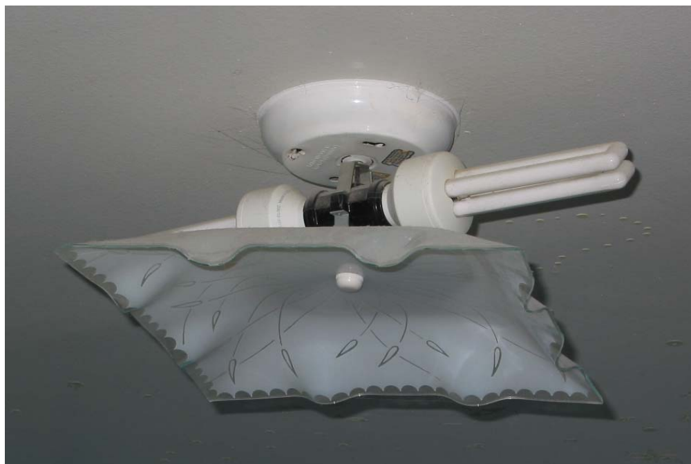
Figure 2. Photograph of compact fluorescent light bulbs installed in an incandescent fixture. The original diffuser for the bulbs was flipped upside down to make room for the longer bulbs. In the inverted configuration, the diffuser is not as attractive, and it is not very effective because the bulbs protrude. This bulb did well in an entry market—appealing to consumers who wanted to conserve energy—and performing very well, but it was not a long-term success. This style of CFL bulb is no longer widely available, most likely for the obvious reason.
