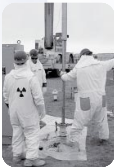
In January 2000, two cranes lifted the 55-foot Corrosion Probe into position over the riser, and operators on the ground helped guide the probe into Hanford Tank AN-105.
