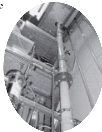
Ion-exchange column loaded with crystalline silicotitanate.
