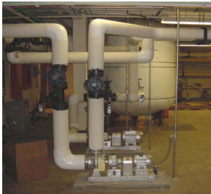
Fig 8: Circulation Pumps and Storage Tank
