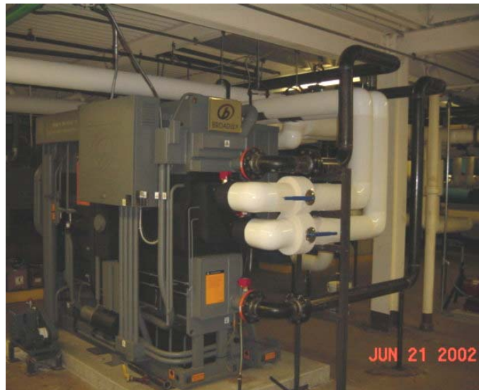
Fig 7: 50-ton Double-Effect Absorption Chiller
