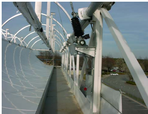
Fig 10: Power Roof™ Receiver Positioning System
