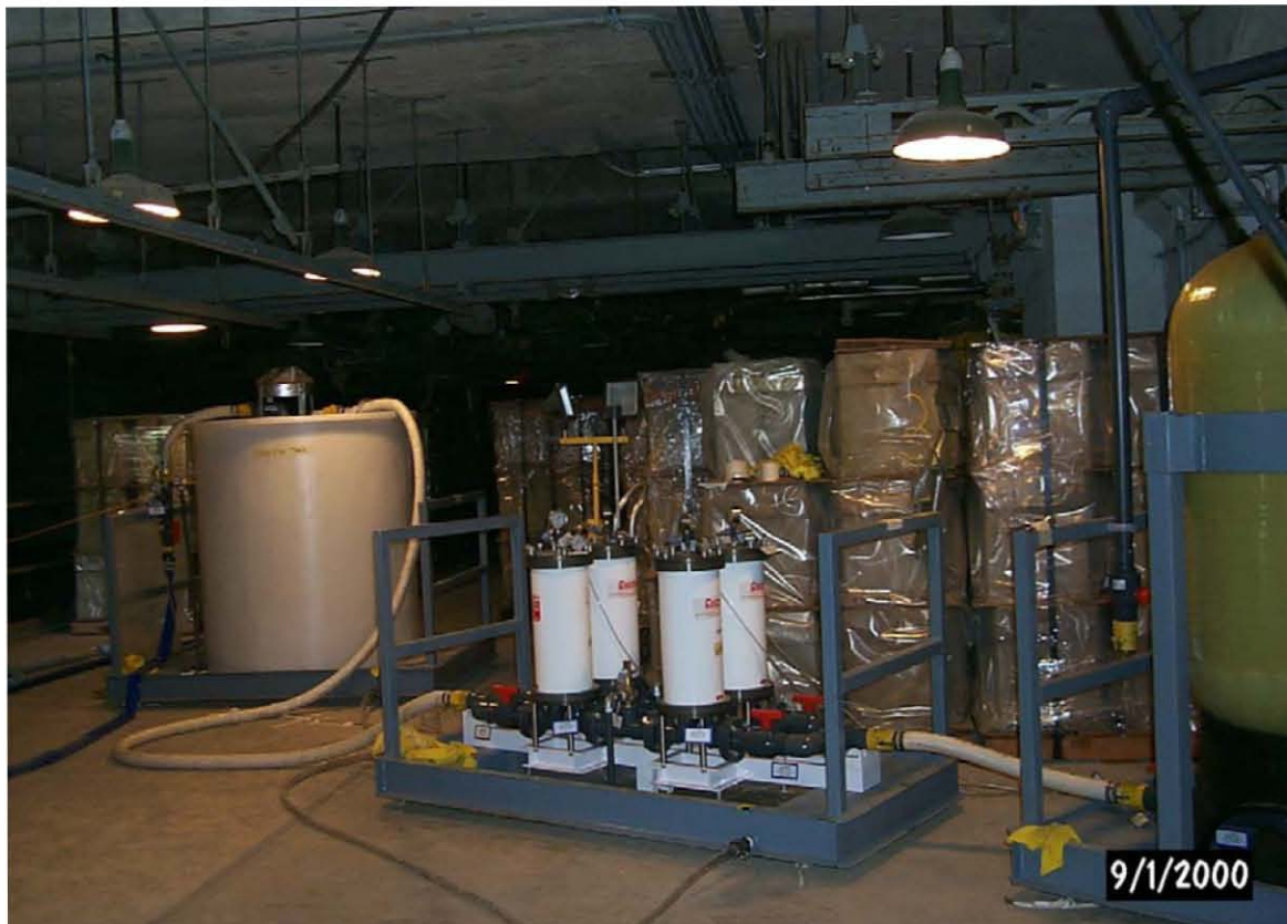
Fig. 1; Graver/Selion System in R-Basin: Activated Carbon Tank to the Right, with the 1 and 5 Micron Filters in the Center, and the CsTreat® Inside the Shielding Tank to the Left
