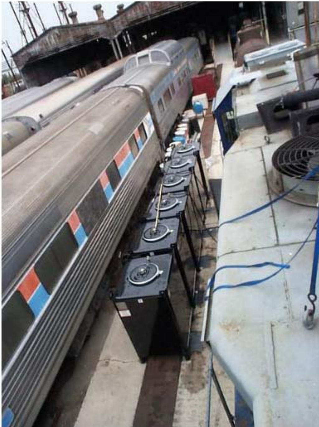
Figure 2. 550-Gallon Fuel Storage Tanks Located Next to Locomotive
